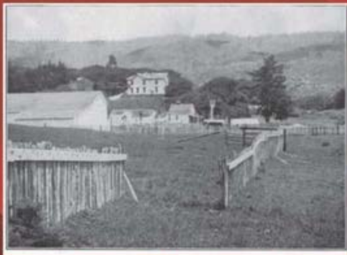
A fence offset by the 1906 earthquake along the San Andreas fault.
